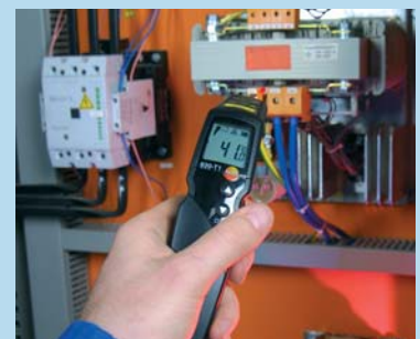
2 mm measurement point for surfaces with a small diameter (testo 830-T3)
