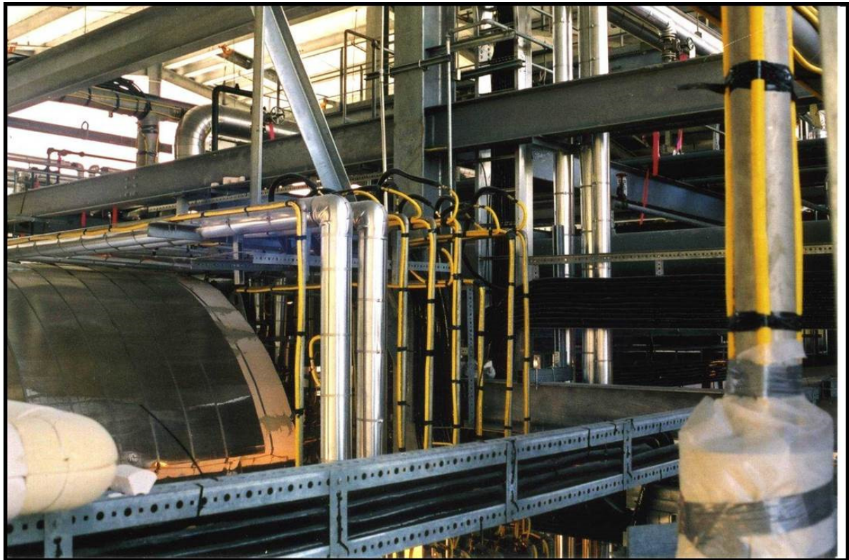
Figure 2: “Safe Trace” installation
